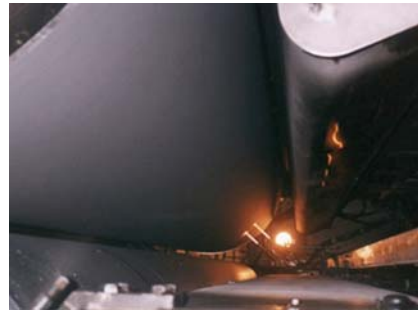
Fig. 3 HVOF spraying of paper machine dryer cylinders on-site (Pikoteknik Oy)
